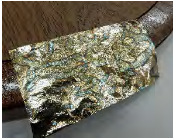
Photo 24 – Laying first piece of metal leaf
